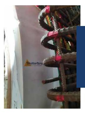
The film can be easily attached to any area of a formwork/shutter to de-activate the setting of wet concrete laitance to expose aggregates for creating a keyed construction joint, for exposing starter bars/couplers and for creating aesthetic decorative finishes. ShutterStrip is ideal where the concrete interface is expected to transfer tensile and shear stress forces.
